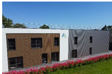
ADVANTELEC Usine de batteries
